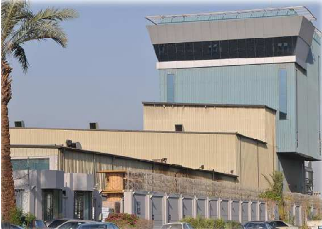
Outside view of the CV-Line at the MV/HV plant
